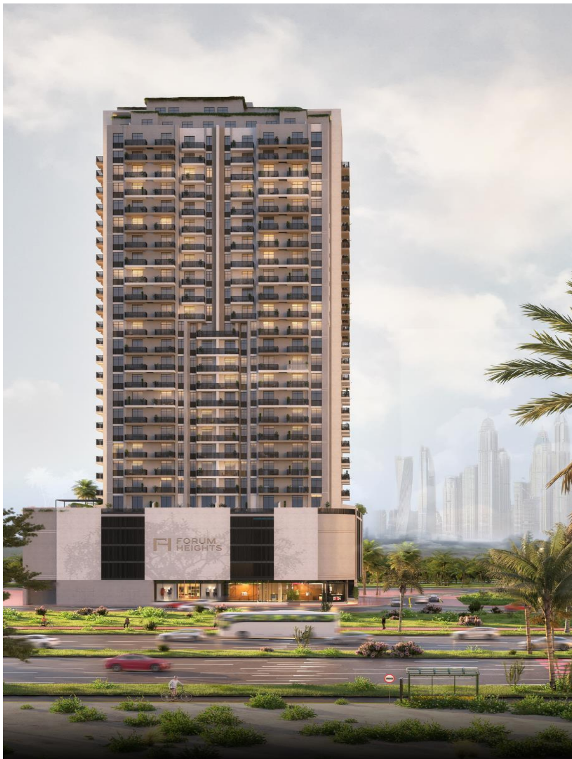
UG+G+4P+24F+R RESIDENTIAL TOWER On Plot No JVT 03G HRA 001, at JVT, Dubai
