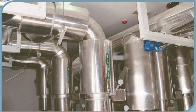
JSS International School @ Al Barsha - Dubai
