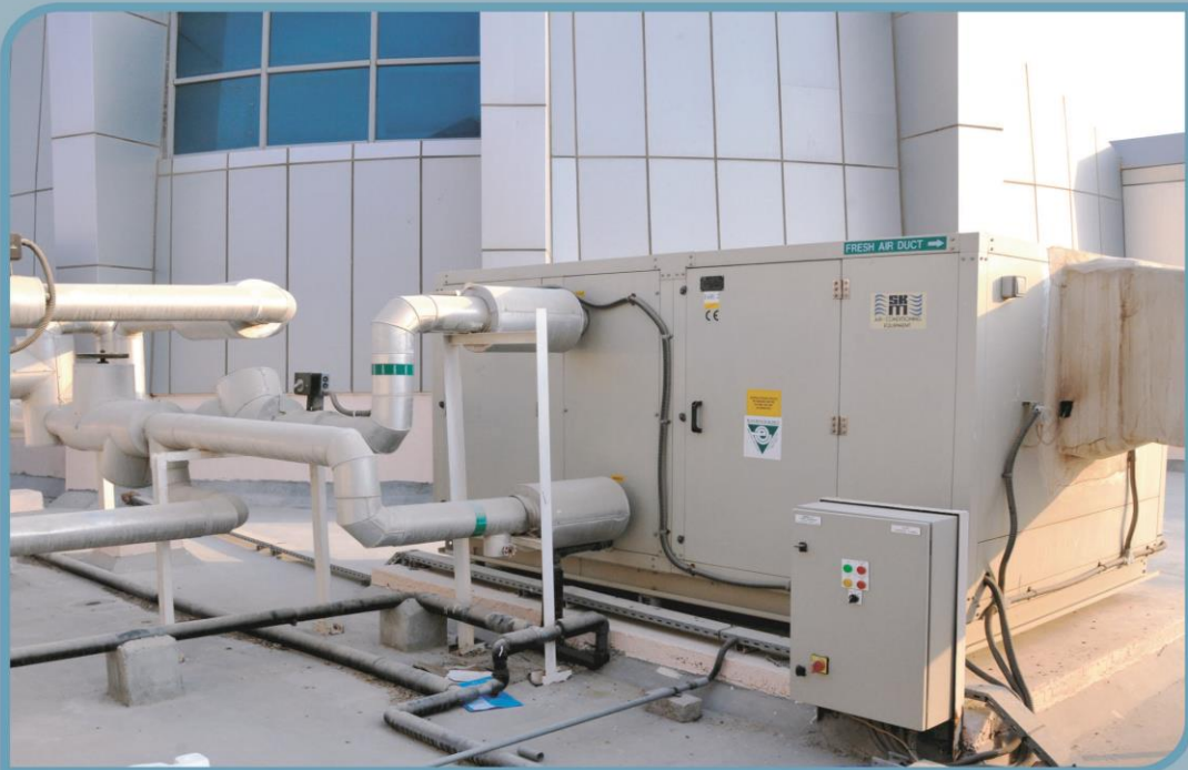
JSS International School @ Al Barsha - Dubai
