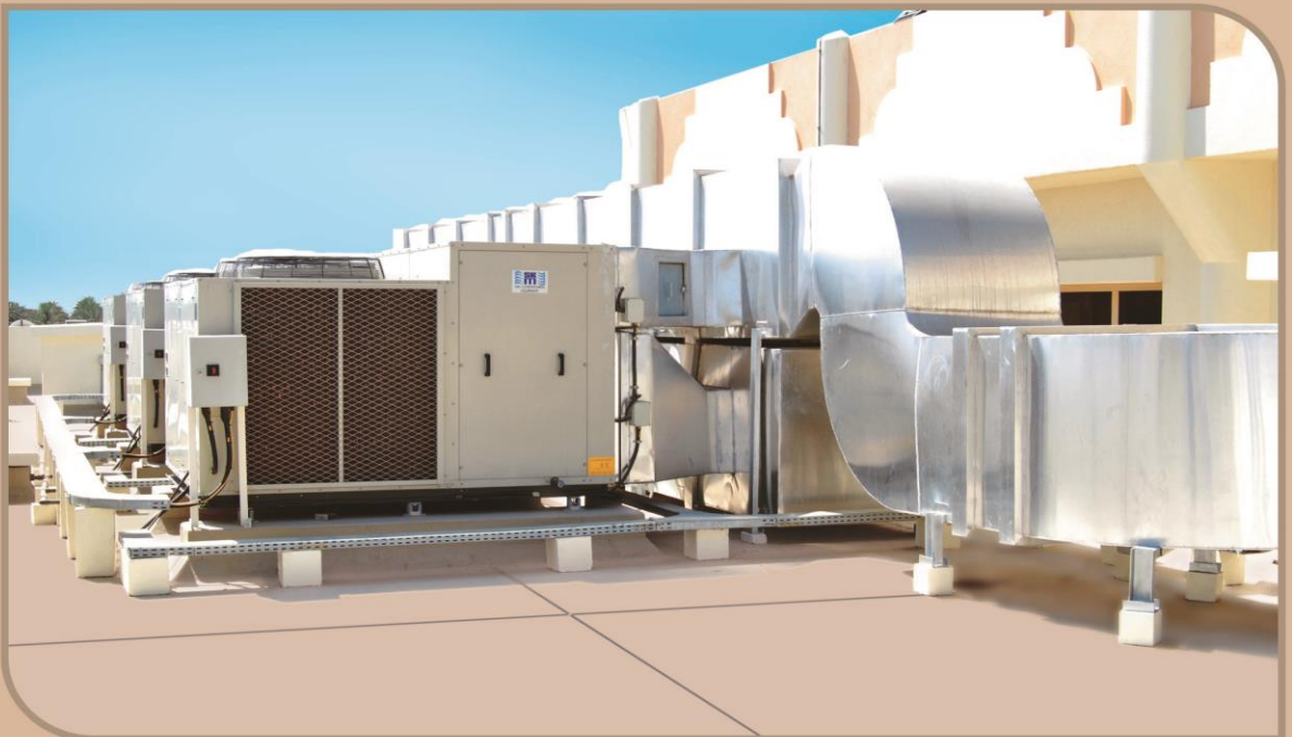
132/11 KV Substation @ Al Dhaid
