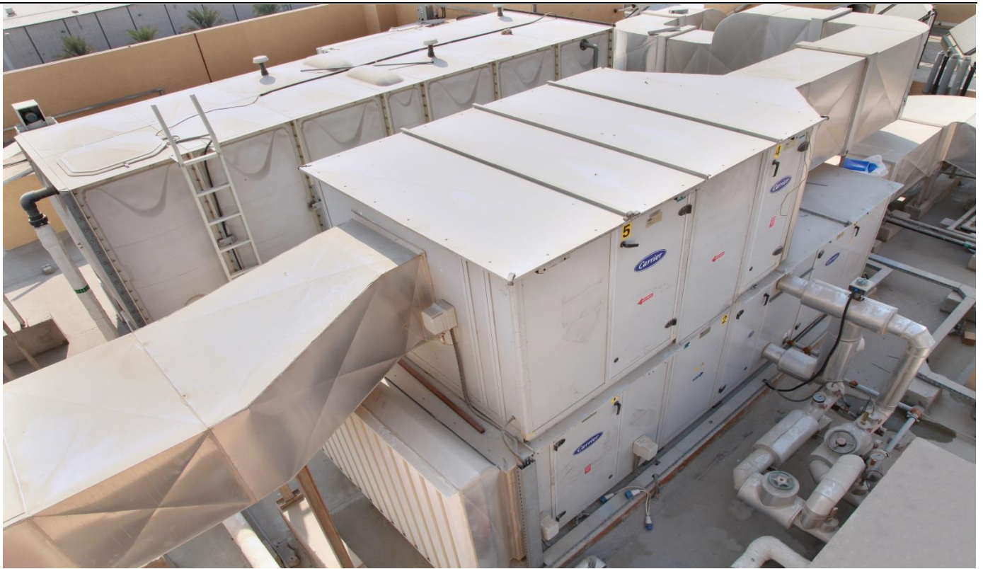
AL FANAR LABOR ACCOMODATION (G+4) AT DIP
