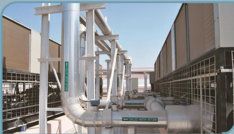
JSS International School @ Al Barsha - Dubai
