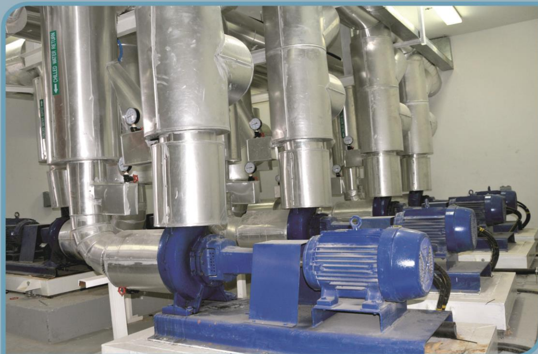
JSS International School @ Al Barsha - Dubai
