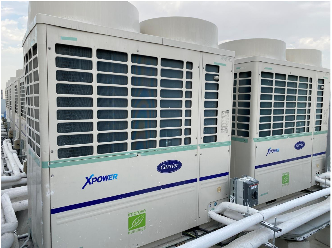
B+G+P+5+R (PENROSE PLACE) RESIDENTIAL BUILDING AT JUMEIRAH VILLAGE CIRCLE
