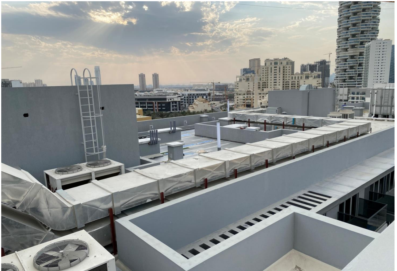
B+G+P+5+R (PENROSE PLACE) RESIDENTIAL BUILDING AT JUMEIRAH VILLAGE CIRCLE
