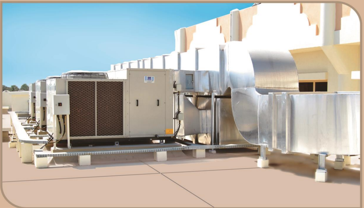
132/11 KV Substation @ Al Dhaid
